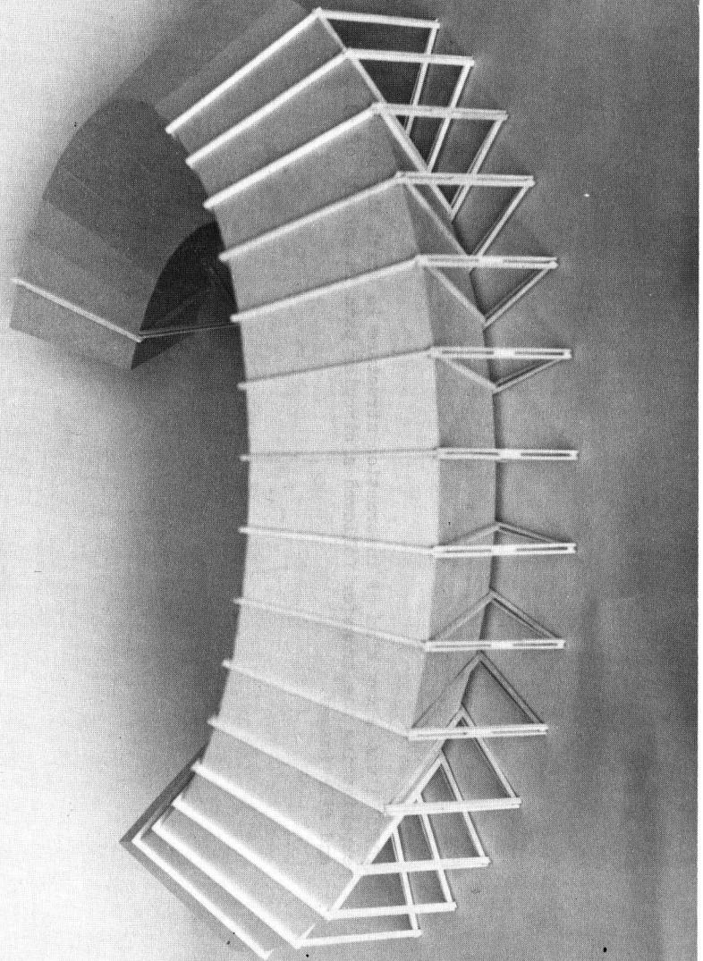
TORUS 1 was constructed of timber and flat panel elements for easy breakdown and shipping.
