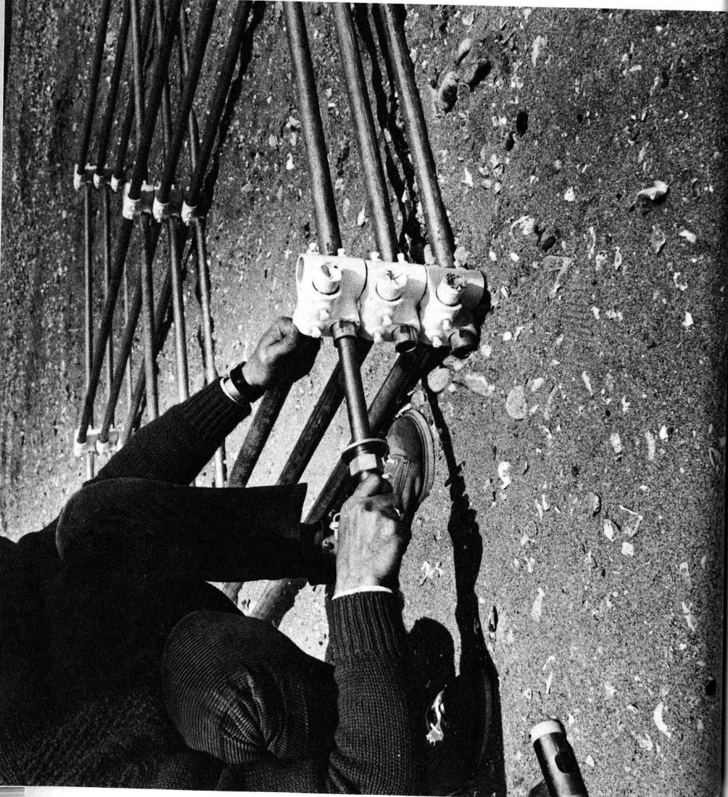
The basis of the MATRIX NETWORK is assembled flat on the ground.
