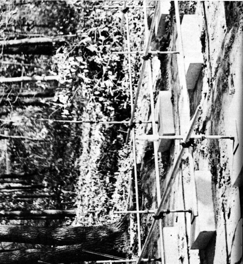
MICROHouses require no conventional foundation which is in keeping with their tradition-breaking form. They are set on pads or feet which are at grade level.
