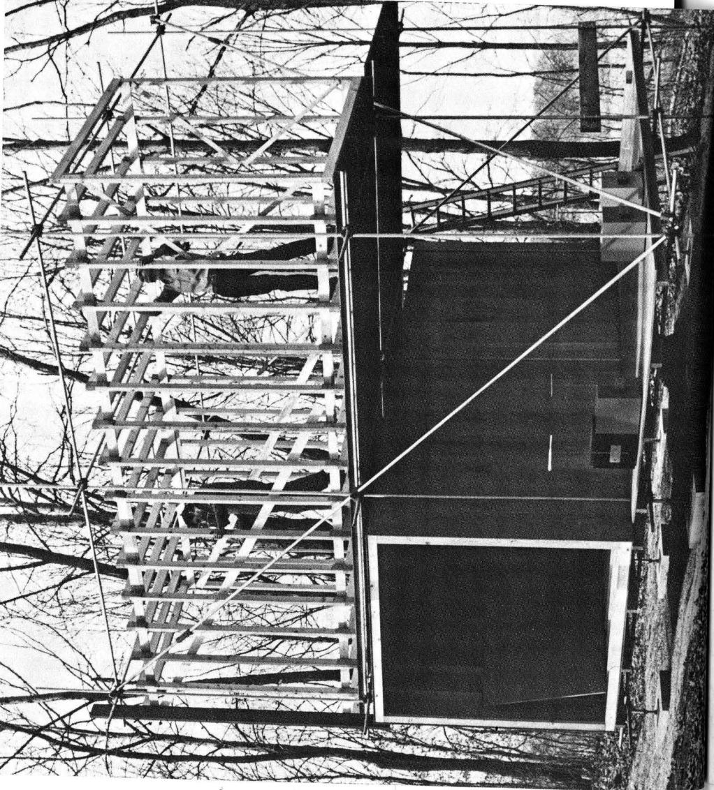
The prototype MICROHOUSE at Groveland under construction. Later versions are completely panelized in plastic or plywood.
