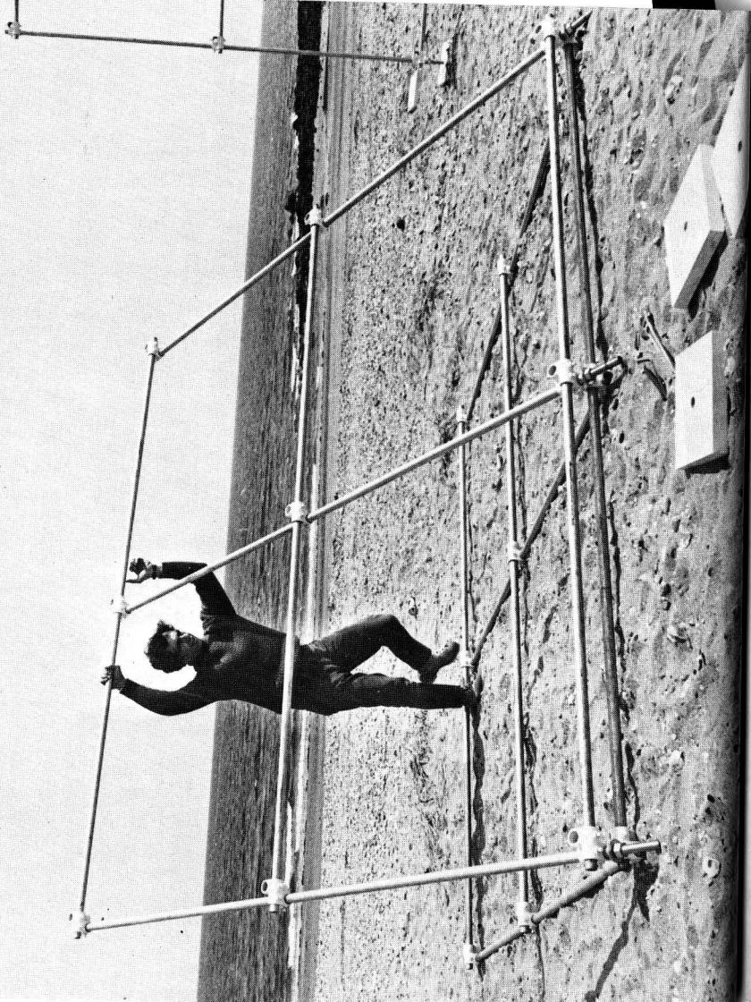
*Actualizing the MATRIX NETWORK.* One of the values intrinsic to this type of structure is the ease with which it can be assembled or broken down for relocation.
