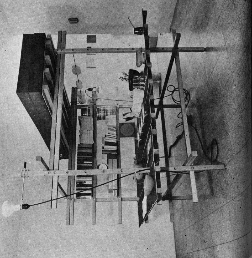
All the members of the unit are 72" long and pack in a case less than 12" square. Easy to move and ship, LIVING STRUCTURES are also simple and inexpensive to produce. Initial cost to the user is a fraction of the aggregate cost for furniture of the old culture.
