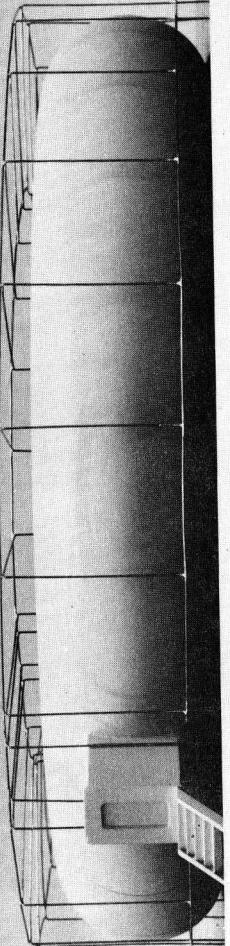
This air supported TORUS 2 is surrounded by a knockdown frame of aluminum tubing used for mounting the projectors. The entry airlock is at left.
