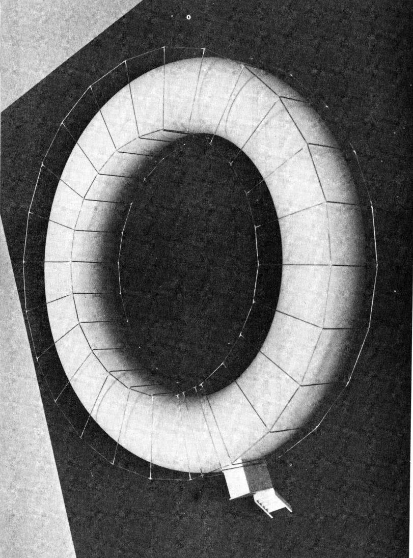
This air-liftable version of the TORUS information structure utilizes an enclosure and projection surface of non-rigid plastic supported by higher interior air pressure.
