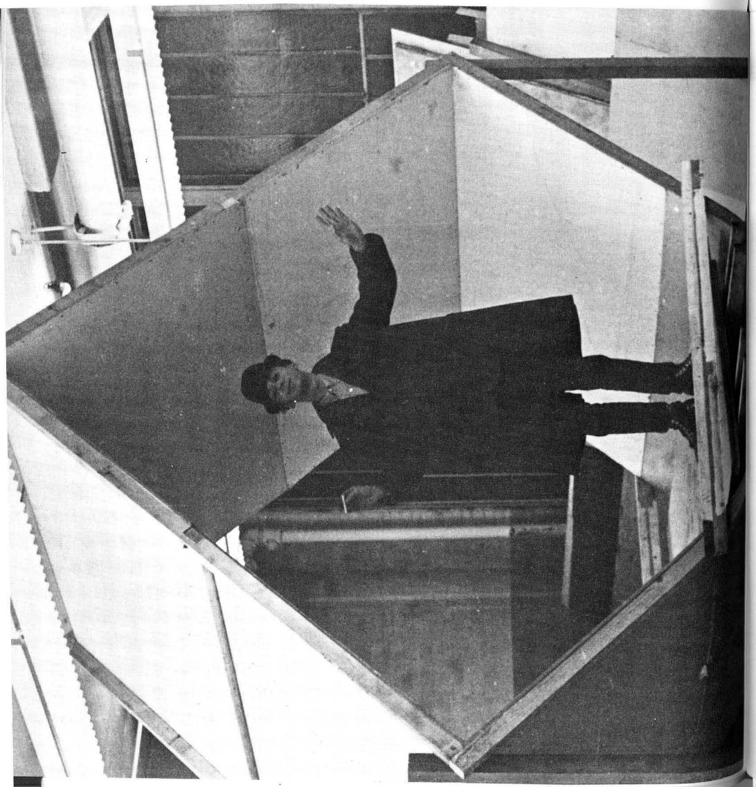
This full-scale cross-section mockup of TORUS 1, built at the Rhode Island School of Design, shows the relationship of the walkway to the four inclined projection surfaces which surround the participants.
