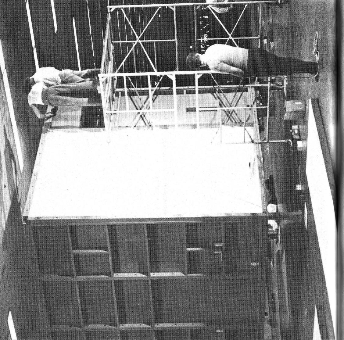
Simple bolted construction was used. Experiment is often impeded by notions from the old fashioned culture which suggest that only elaborate and over-complicated technology can produce new and useful ideas.
