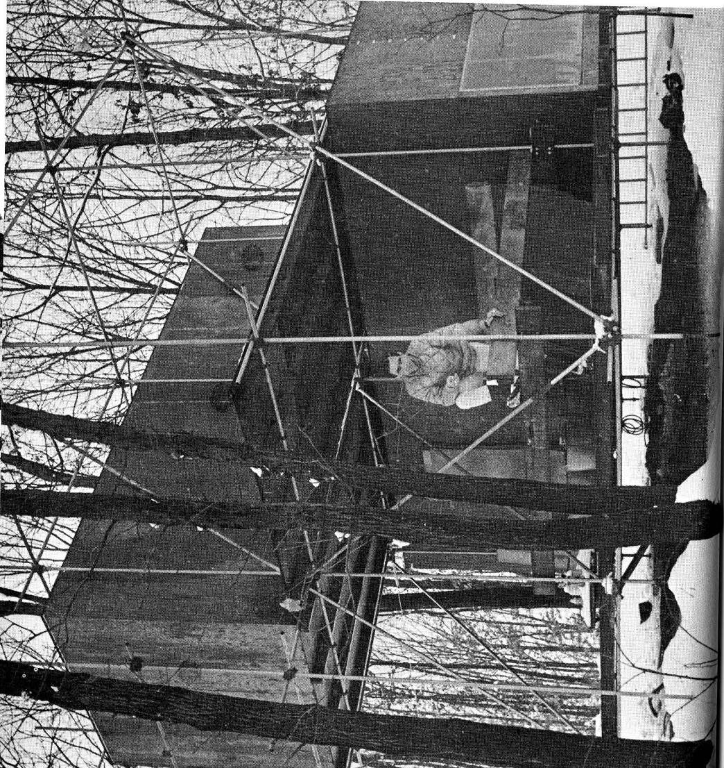
Despite the fragile appearance, the NETWORK is sturdy having survived winds of 80 mph. The closed volumes are insulated and comfortable in temperatures of -20 degrees F.
