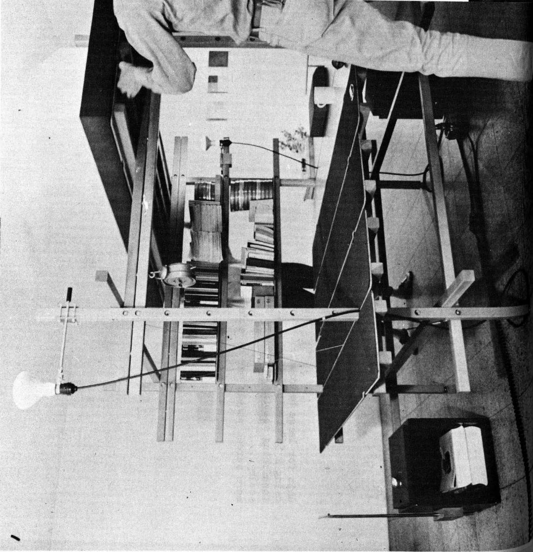
The Chicago LIVING STRUCTURE 6 x 6 consists of a wooden frame of members  $1\frac{1}{2}$ " square bolted in the non-collapsing joint at the corners.
